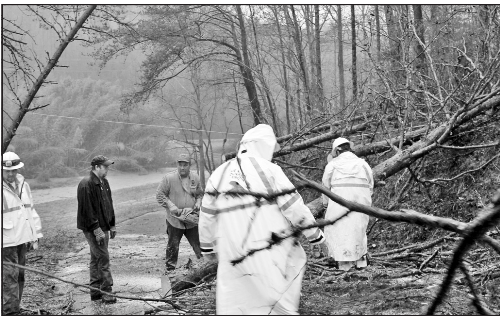
EMC crews work to clear downed trees to allow them to replace a twisted off power pole off Georgia 515 in Union County. Mother Nature kept the crews busy for 27 hours, Wednesday into Thursday. Photo/Libby Shook
